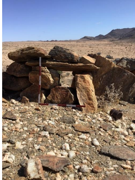
Figure 18: Typical UDF rifle loophole. Note that the resting position is approximately 20cm above ground level.
